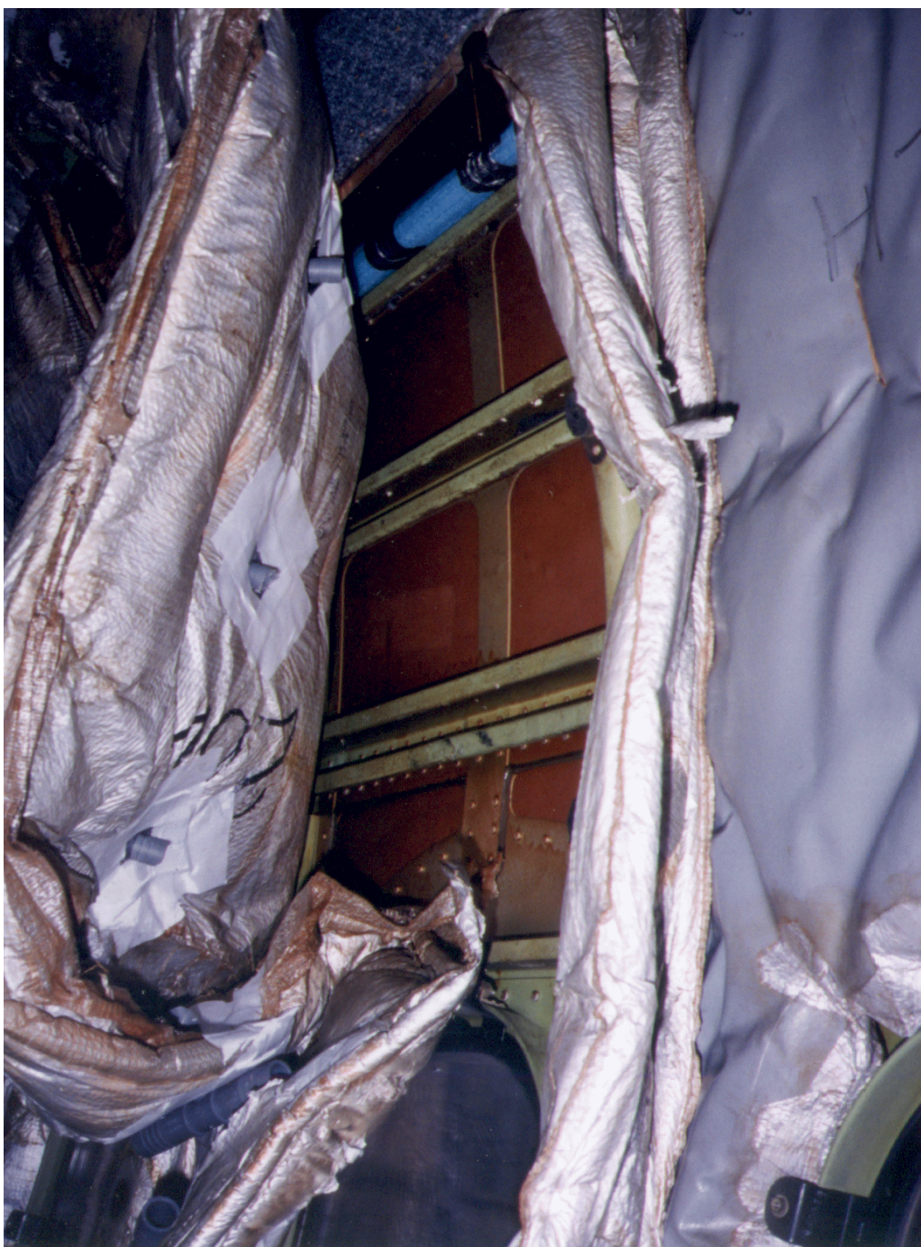
Figure B.3 View of 3/4"ID PVC injection air tubes, 1/4" and 3/16" ID PVC pressure and VOC sampling tubes between the B737 cabin insulation and liner
