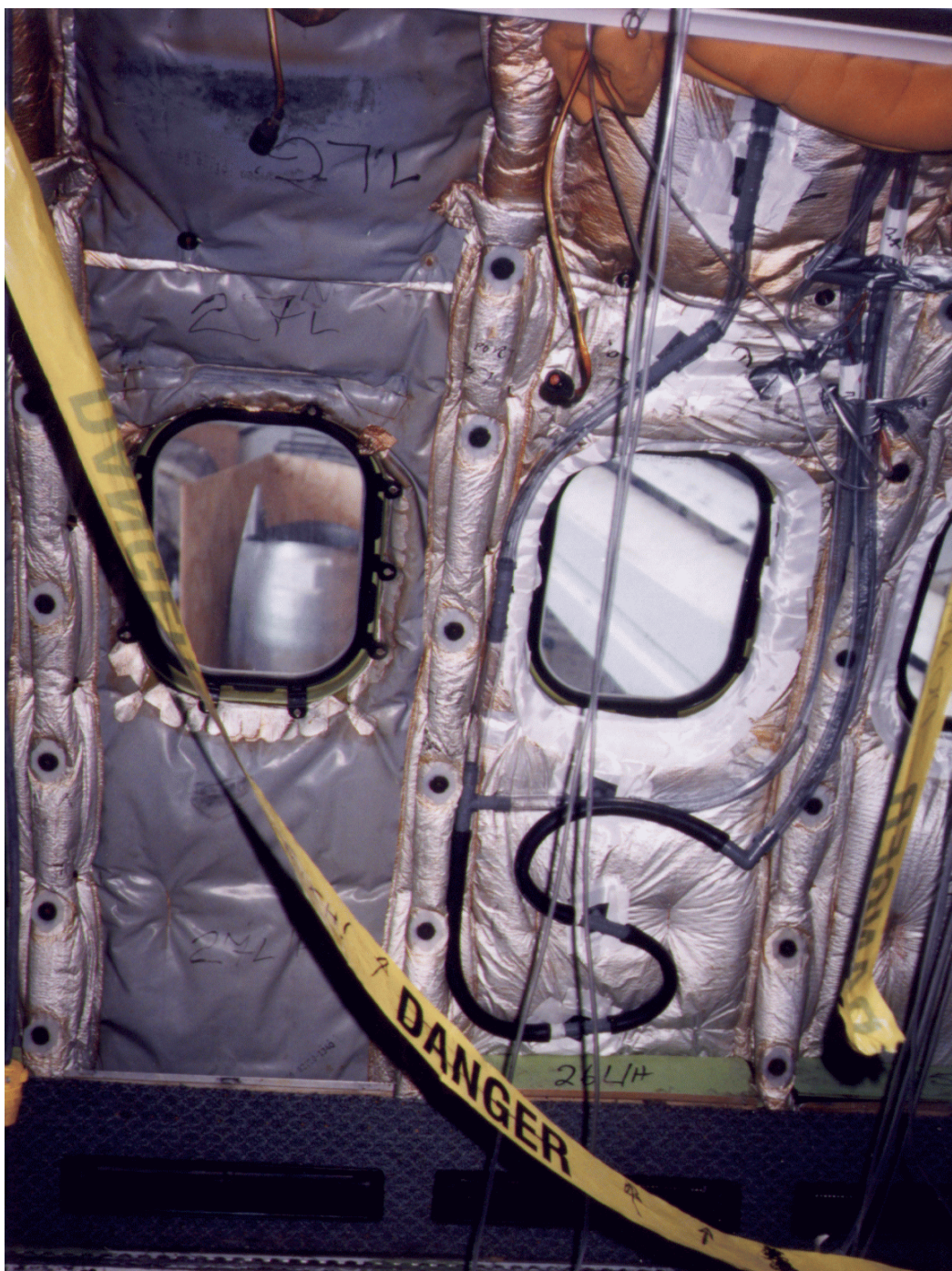
Figure B.2 View of 3/4"ID PVC injection tubing behind the B737 cabin insulation
